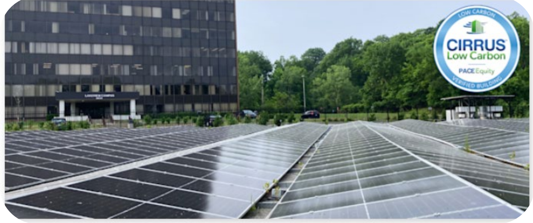
Euclid Office Building Euclid, OH
